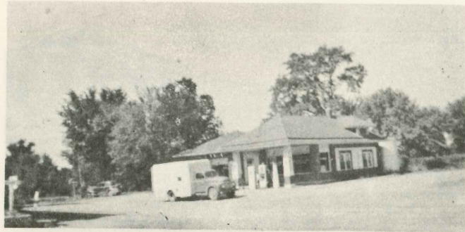
Stade Service Station and Cafe.
