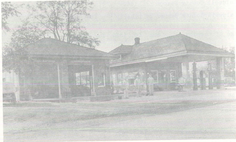
ELMER STRATTON FLOYD STRATTON RAYMOND LEWELLEN ABOUT 1935 (HOME OF AMBULANCE AND HEALTH OFFICE, TODAY)
